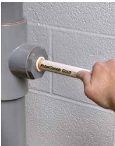
Installation of C-PVC pipes
